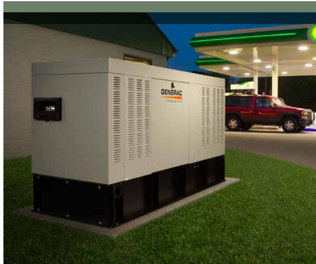
Local codes, property restrictions or your unique power needs might mean moving up to a permanently installed solution. This is known as automatic standby power, and it's the choice of most businesses. As the name implies, these power systems start automatically when utility power is interrupted, and shut down automatically when utility power returns. Choose from diesel, LP, natural gas or bi-fuel systems.
